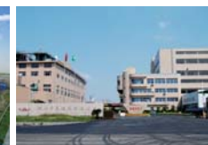
TBR Plant in Xiasha
